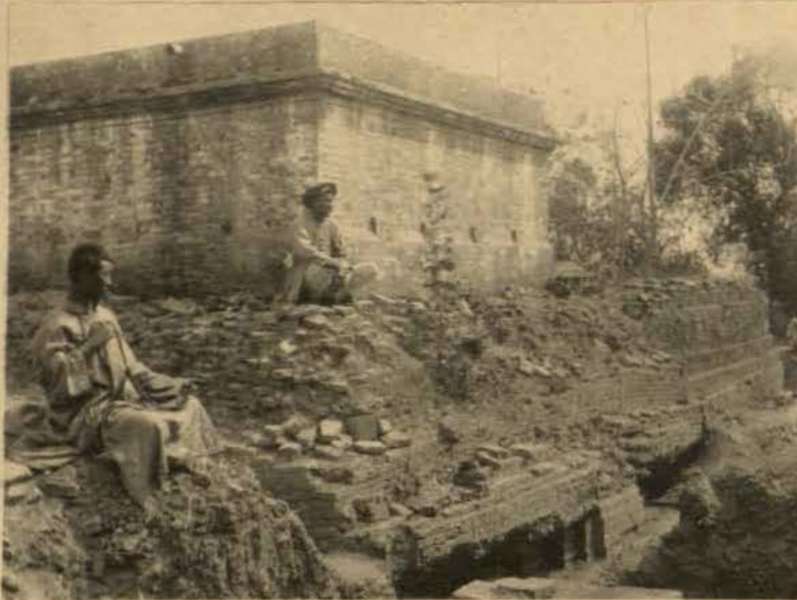
RUMON-DEI VIEW OF MAYA-DEVIES TEMPLE. SHOWING FOUR PERIODS OF BUILDINGS FROM S.W.
